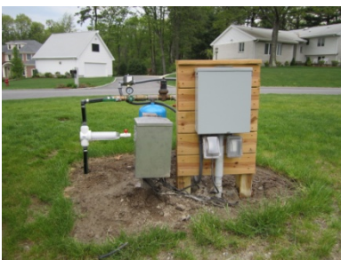
Well, Tank, Filter & Electrical Components hidden under Artificial Rock(to be landscaped later)
